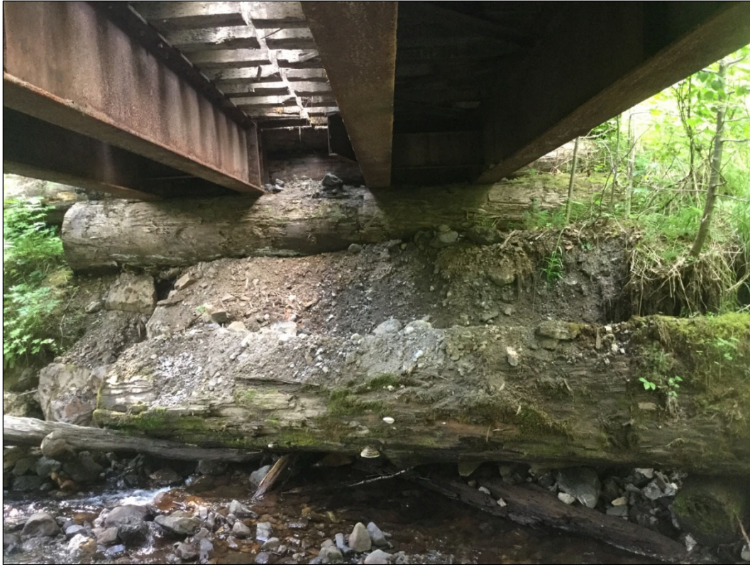
Figure 3.—River-right bridge abutment with collapsed log at waypoint 938.
